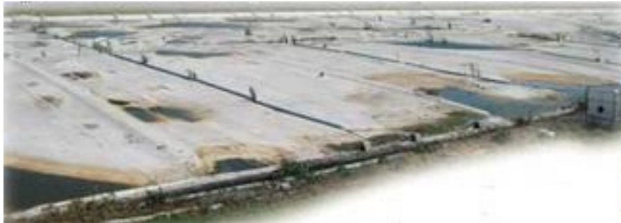
Casco's 20-year-old cover prior to replacement
