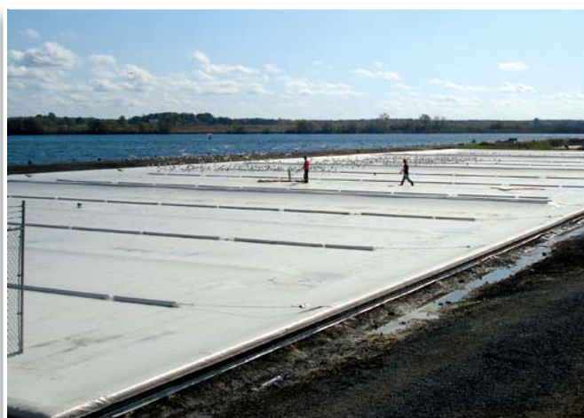
Casco's new GTI floating geomembrane cover.
