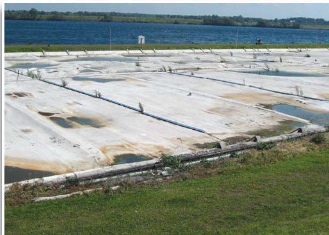
Casco's 20-year-old cover prior to replacement.
